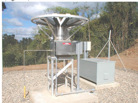
Figure 6: 500 Watt TEG on a natural gas pipeline in Peru [Courtesy LeSage, Global Thermoelectric]
